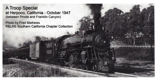
Santa Fe Number 3450 is a Hudson type steam locomotive designed for high-speed passenger service. It was the first of ten similar coal burning 4-6-4 wheel arrangement locomotives built for Santa Fe in 1927 at a cost of \$73,735,60.
